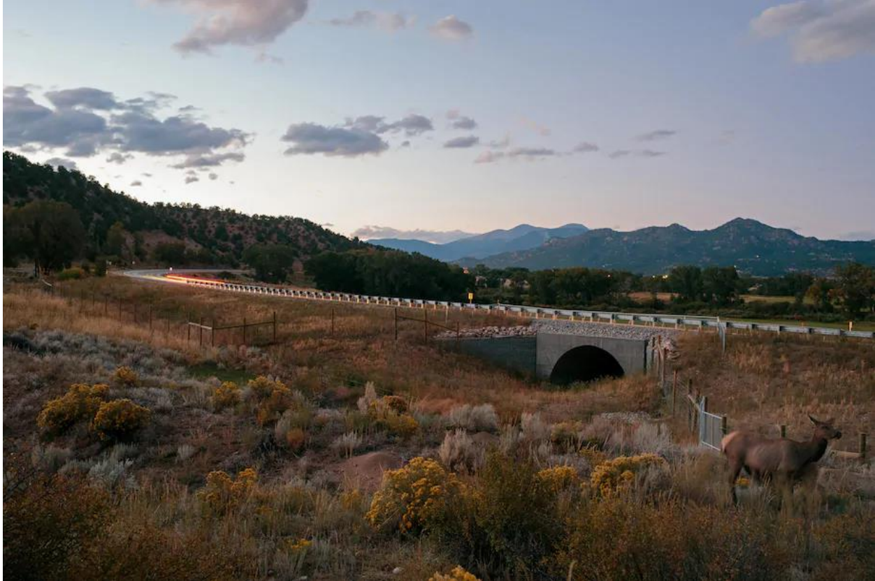
Two elk stand by the road as traffic moves over a large underground crossing structure that serves as part of a Colorado wildlife corridor. (Matthew Staver/For The Washington Post)
