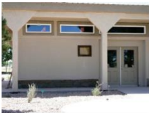
Straw Bale Structure & Demonstration Garden – Partners: CCSD, DAQEM, Mesquite / Overton
